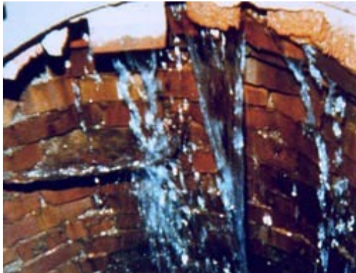
Storm water entering into the sewer system from a manhole, at left, and from a defect inside a pipe, at right.
