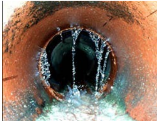
Storm water entering into the sewer system from a manhole, at left, and from a defect inside a pipe, at right.
